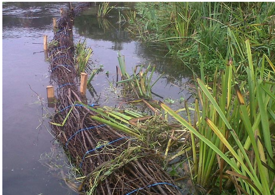
Figure 13. Example of brushwood bundle used to prevent bank erosion
